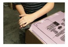
25. Use a sanding block to smooth the edges of the hardboard and foam.
