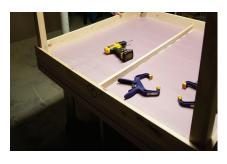
10. Add a 1x2 under the foam across the center. This will keep the foam from possibly sagging and, once drilled (Step 11) will provide support for wiring.
