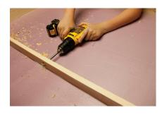
11. Use a 1/2" spade bit to drill several holes in the 1x2 support. You can later run your wires through the holes to keep them from dangling.
