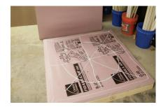
6. Attach the second foam insulation board to the top of the first with a generous amount of foam adhesive.
