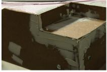
31. Use Bondo All-Purpose Putty to cover any nail holes and fill in any gaps in the hardboard. Sand and paint when dry. Use caulk to
