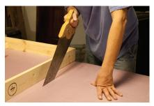
4. Use a saw to cut the foam insulation board in half, making two 4'x4' pieces. Make sure these pieces are the same size as the
