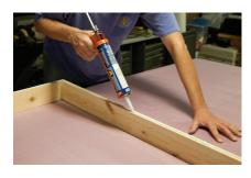
5. Use the foam board adhesive to attach one of the insulation boards to the frame.
